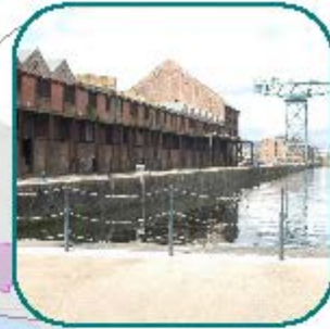
James Watt Warehouses, Greenock
