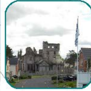
Former Broadfield Hospital, Port Glasgow
