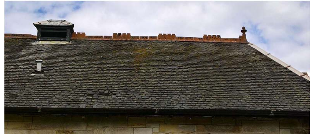
Slates missing and slipped
