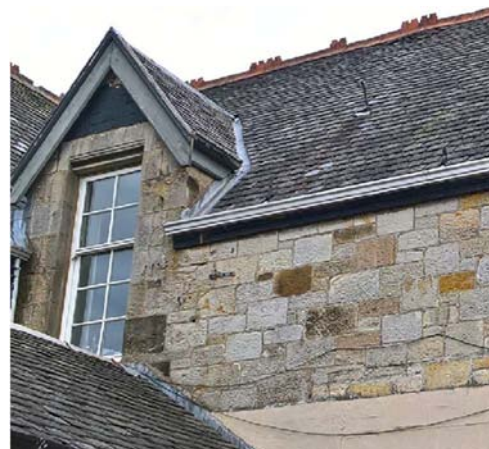
Replacement guttering in aluminium
