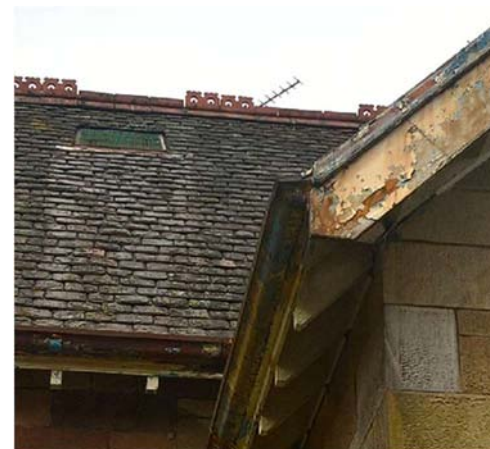
Blocked and corroded guttering
