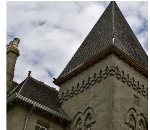
Roof flashing missing - Spanish slates in use
