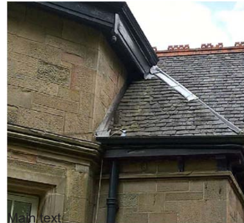
Overlaid zinc flashing over original lead
