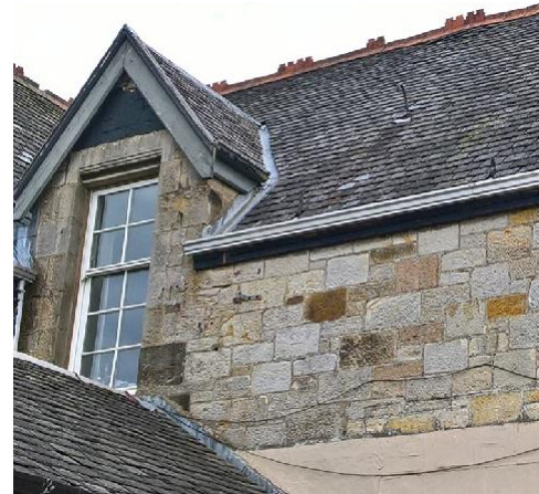
Replacement guttering in aluminium
