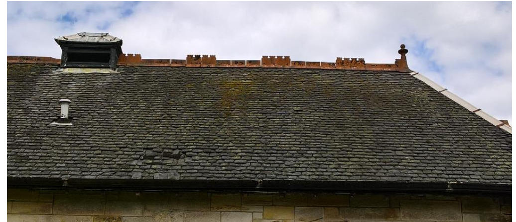
Slates missing and slipped
