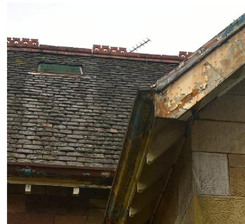
Blocked and corroded guttering
