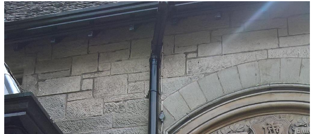
PVC downpipes in use
