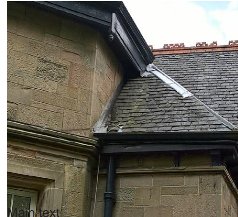
Overlaid zinc flashing over original lead
