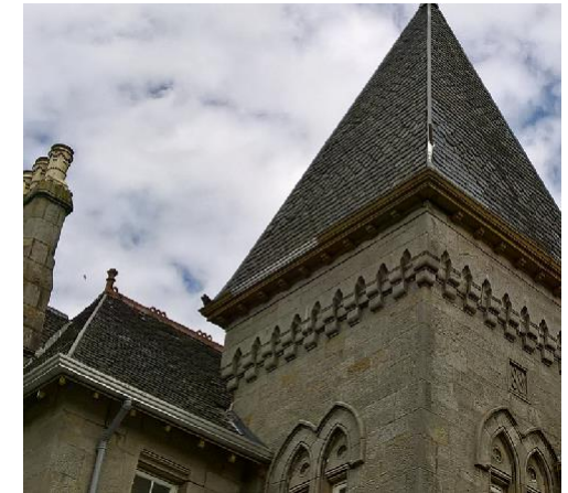
Roof flashing missing - Spanish slates in use
