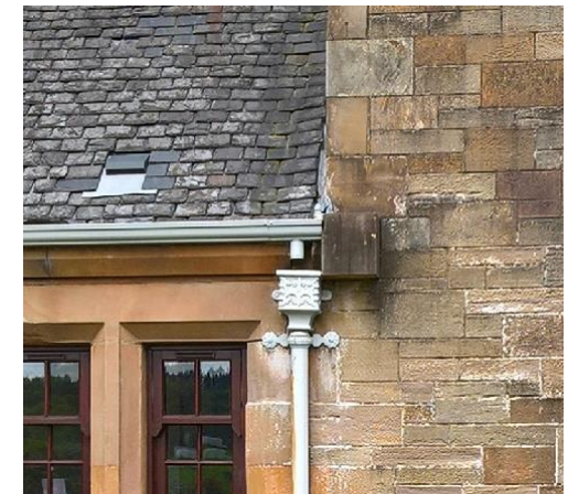
Original cast iron fittings at Glenfarg
