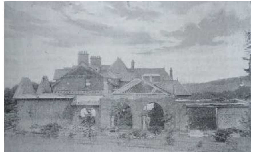
Executive Buildings – after the fire.
