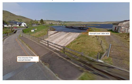
Photo 7: Overspill of the compensation reservoir
