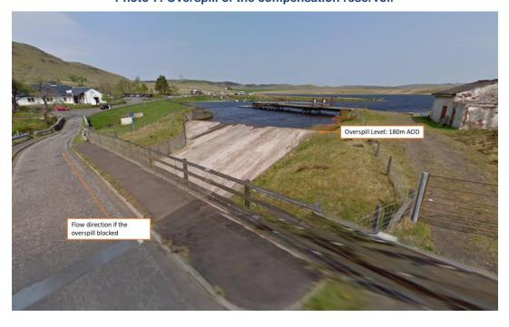
Photo 7: Overspill of the compensation reservoir
