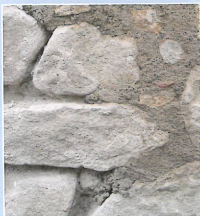
Modern lime mortar pointing, Scottish Lime Centre, Charlestown, Fife. The use of lime allows the wall to 'breathe'. Traditionally, most rubble walls had lime slaistered, or buttered, over the joint to achieve a fairly smooth finish that would erode with time. Where pointing does not alter the character of a listed building it would not normally require consent.
