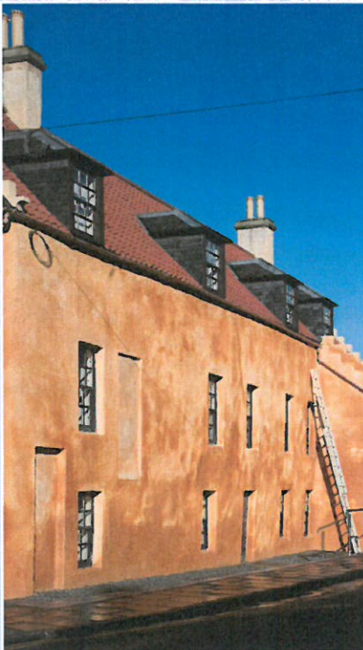
Dymock's Buildings (late 17th century), Bo'ness, were restored by the National Trust for Scotland in 2004. A cement render was removed, the archaeology of the wall recorded, and then a lime harl and limewash were applied. Evidence of former openings remains visible. © N. Haynes.
